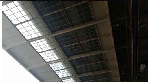
Hanger 4 Door- Side C
