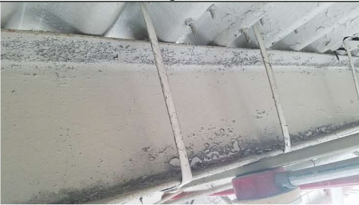
Hanger 4 Ceiling Braces
