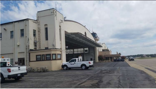
Building - Side C
