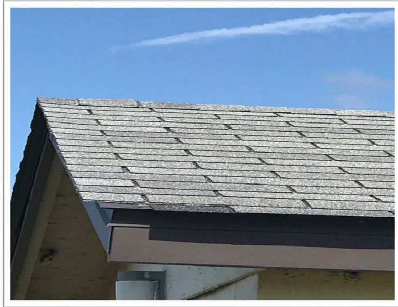
Roofing Material was found not to contain Asbestos
