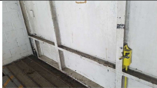
Hanger 4 Wall A
