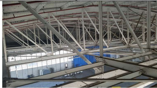
Hanger 4 Ceiling Braces
