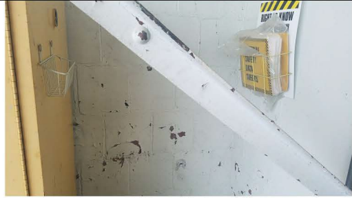
Hanger 5 Block Wall and Brace
