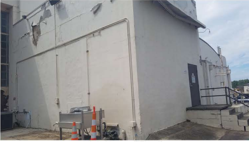
Building - Side A
