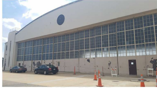
Building - Side A Left
