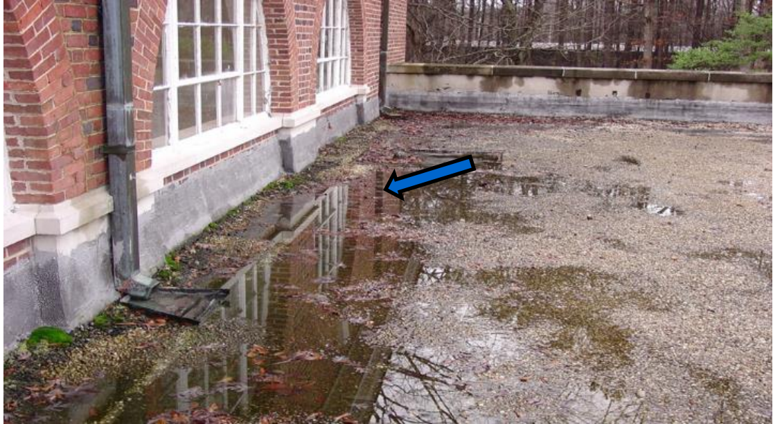
Picture 1 – Standing water must evaporate within 48 hours
