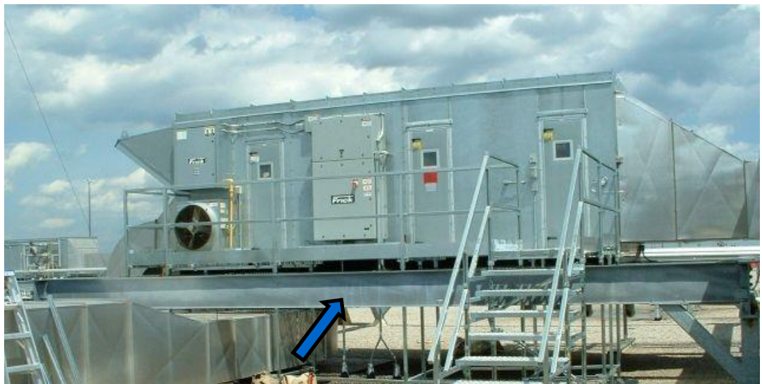
Picture 5 – Mechanical platform or frame
