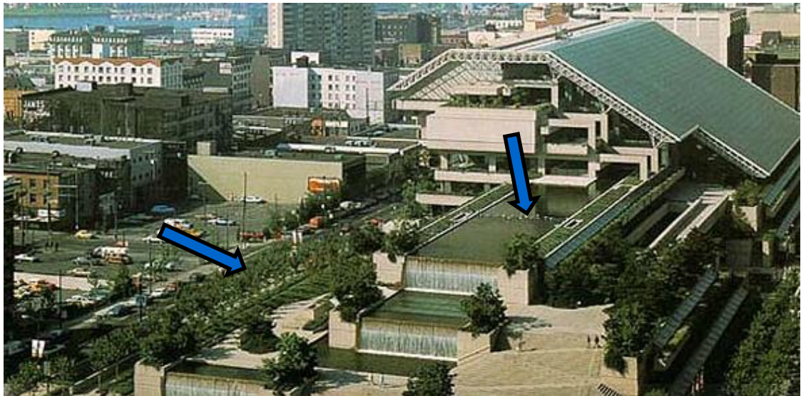
Picture 2 – Garden, plaza, walkway, water feature etc. are roofs of the building
