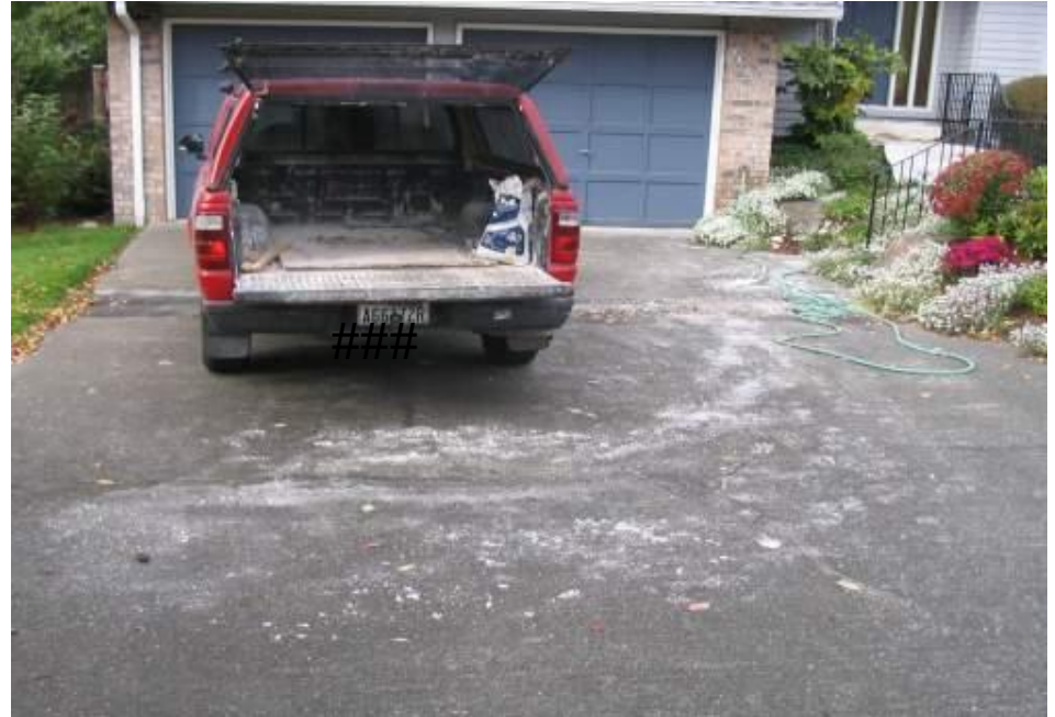
Uncontrolled popcorn ceiling removal job
