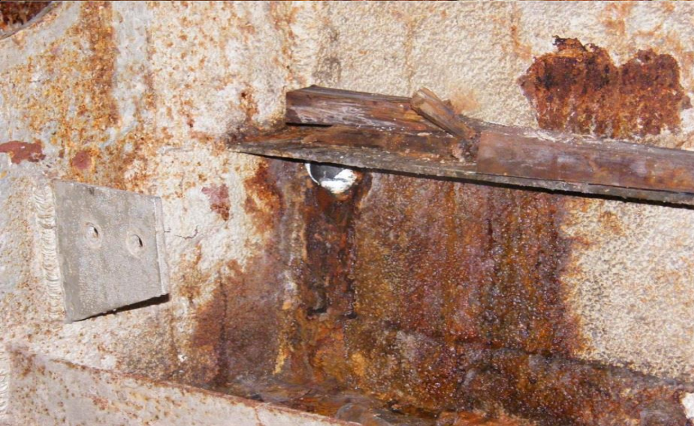
DCR – USS Battleship - Steel hull plating shows excessive corrosion. Battleship is now leaking around hull plating rivets and recent hull surveys indicate hull thicknesses of less than 0.1 inches.
