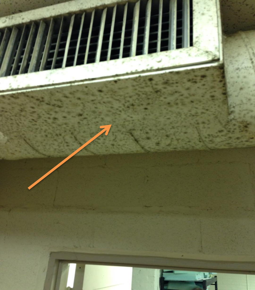
DHHS – Black Mtn. Neuro-Medical Treatment – Moldy ducts.
