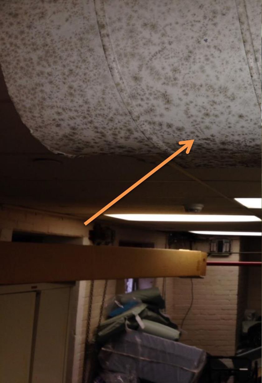
DHHS – Black Mtn. Neuro-Medical Treatment – Moldy ducts.
